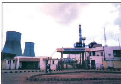
Fig 3.10: A view of a Thermal Power Station
